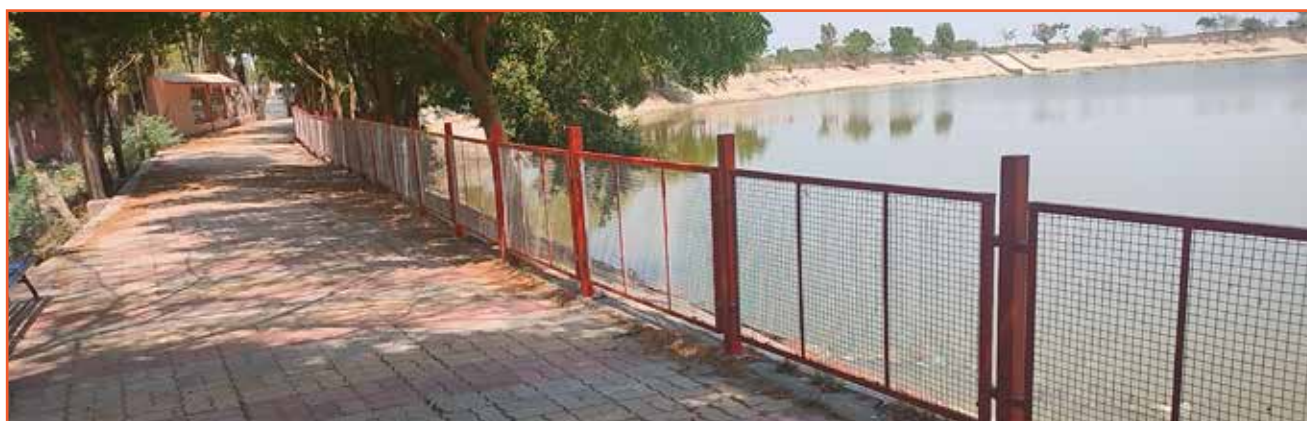
Safety grill installed at the pond in Rahiyad village to help ensure safer surroundings for local residents.
