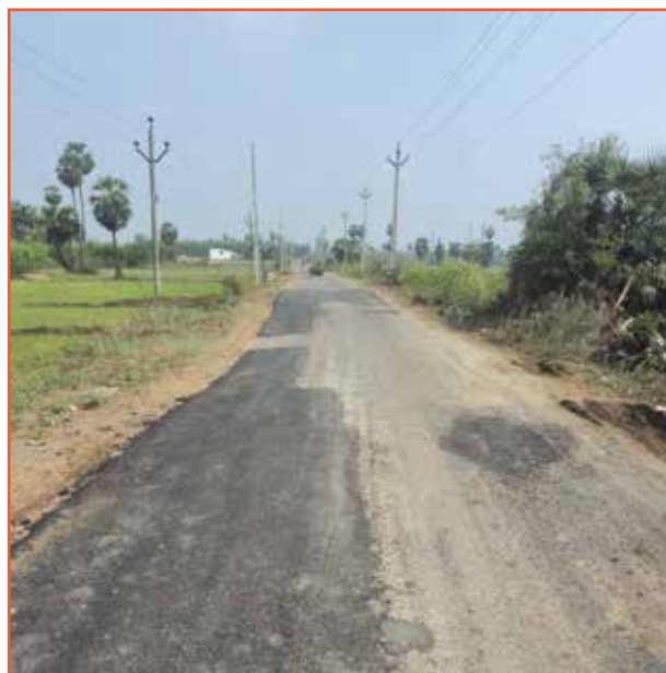
Road repair done in Srikakulam to improve accessibility, safety, and everyday comfort for residents.
