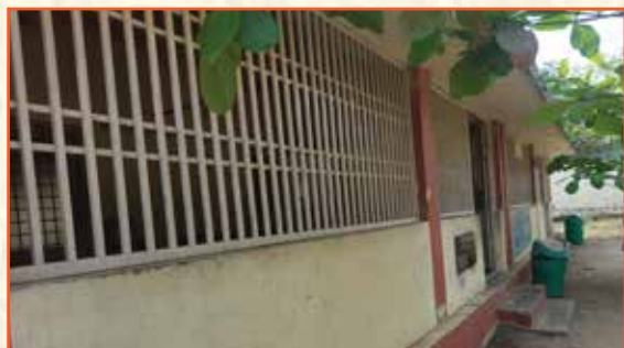
Installation of safety grills at a school in Srikulam to enhance student protection.
